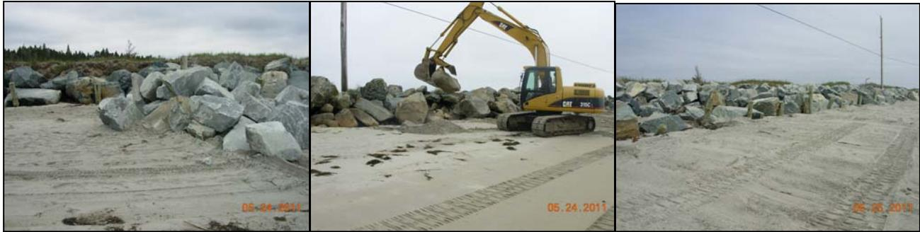
Left: The first load of rock is delivered (note the exposure of the dunes in the rear). Middle: Rocks being individually placed into the cribwork. Right: The finished product! *All photos courtesy of Mary Fulleman*
